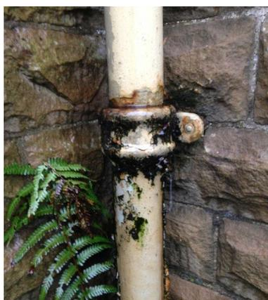
The fixings for downpipes and gutters should be checked as they can work loose. Metal fittings may corrode and cause damage to adjacent masonry or render. Any sign of movement or corrosion should be noted and remedial action taken before further damage occurs. Staining or algae around joints are clues that the connection may be faulty.
