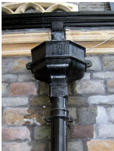
Cold weather can cause severe damage to rainwater goods so it is especially worth while checking for signs of damage during the winter. If gutters or downpipes are blocked, water can easily become trapped and will expand as it freezes. The expansion of trapped water is sufficient to cause downpipes to crack or shatter allowing water to saturate the wall. Look for any signs of splits or cracks and have any broken sections replaced as soon as possible.
