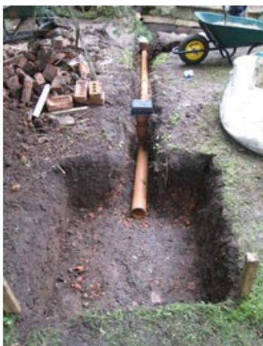
Soakaways are a type of 'infiltration device' - a way of dispersing surface water in situations where it is impractical or impossible to make a connection to the public sewer system.
