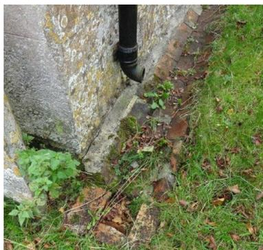
Some buildings will have a perimeter drainage channel or ground gutter running around the building. It is not ideal to have hard surfaces such as brick, stone flags, tarmac or concrete laid against the edge of the building as water tends to splash back onto the wall surface keeping it permanently saturated and encouraging the growth of algae and moss.
